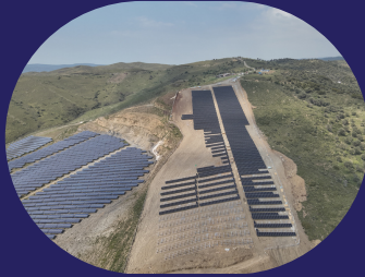
POINT SEREİHİSAR 2.4MWp
